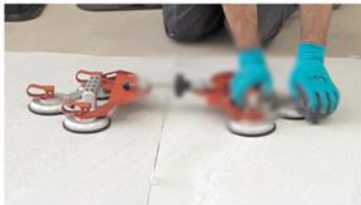
Special device for the plate's pulling over
